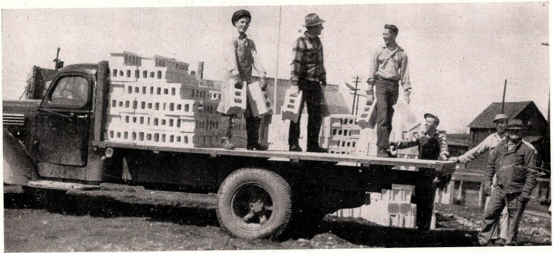
SOME OF THE FIRST CINDER BLOCKS
