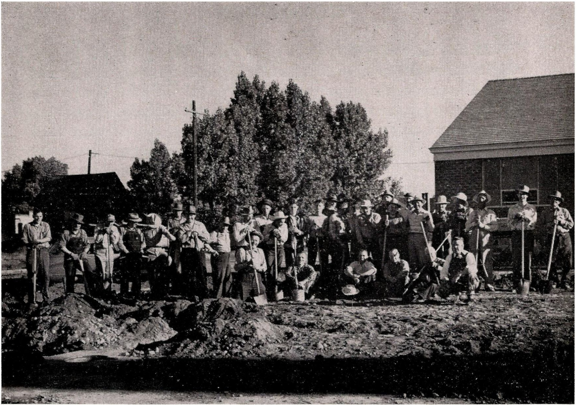
A TYPICAL DONATION WORK CREW. THIS CREW INSTALLED THE SPRINKLING SYSTEM.
